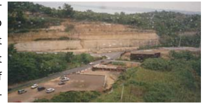
PR-115, Guayabo River Bridge, Aguada, Puerto Rico, looking north
