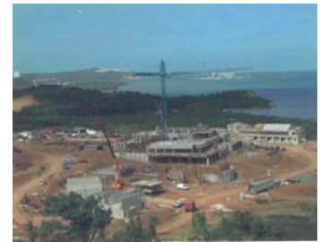
Aerial construction progress photo, Cayo Largo Hotel & Resort, Fajardo, Puerto Rico
