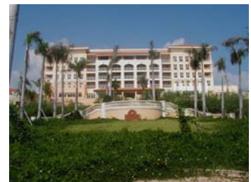
Western Elevation, Cayo Largo Hotel & Resort construction, Fajardo, Puerto Rico
