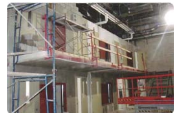
Cell pod construction at Merrimack Jail Facility, Boscawen, N.H.
